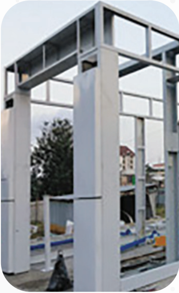
hot dip galvanized frames
